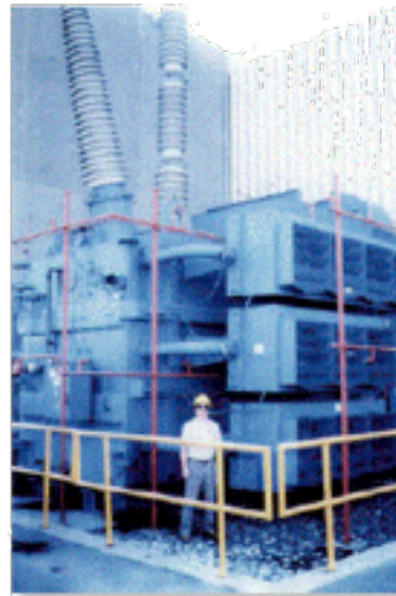
PJM Public Service Step Up Transformer
